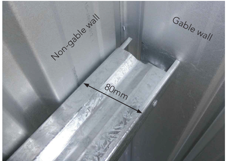
Bracing installed on the non-gable wall between the wall and a portal frame.
