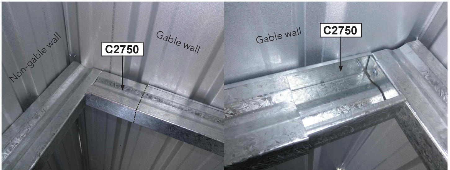
Previously installed wall bracing on the left and new gable wall bracing on the right.
