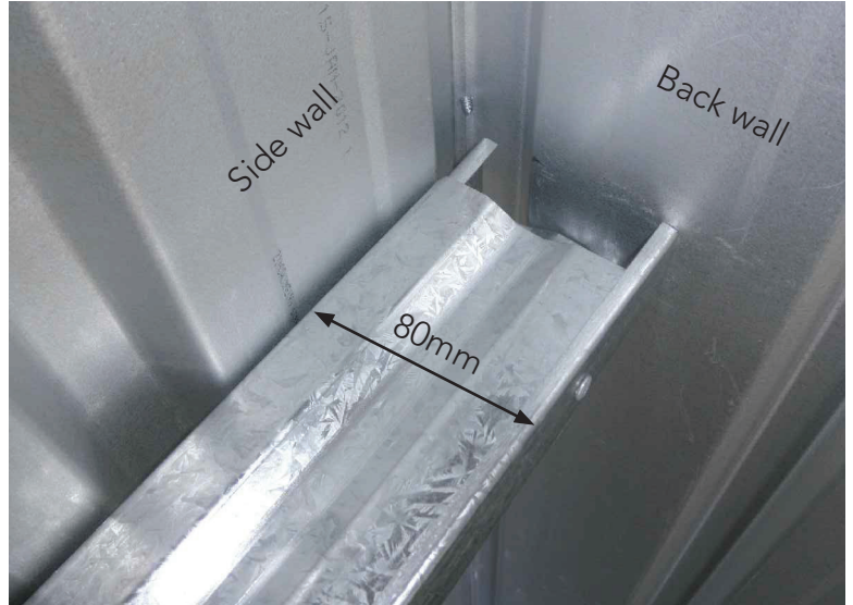
Bracing installed on the side wall.
