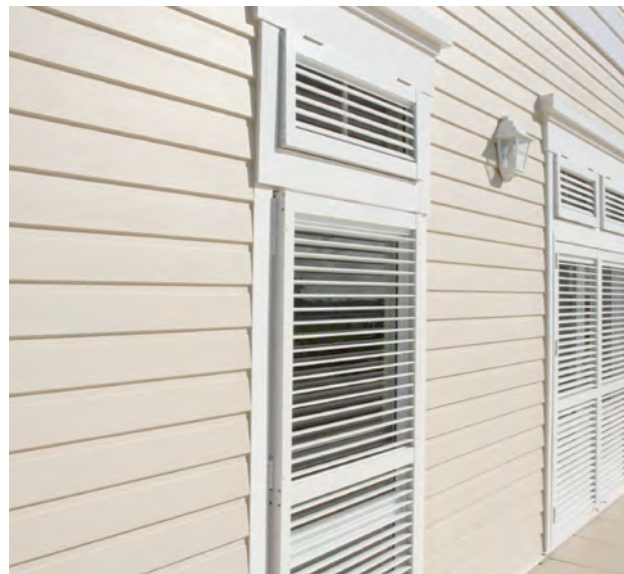
PrimeLine™ Newport Weatherboard 9mm thick Grooved for a deeper shadow line.
