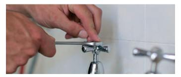
Using a spanner, take off the tap's cover to remove the handle. Some taps may have a small screw under the handle, that can be removed with an allen key.
