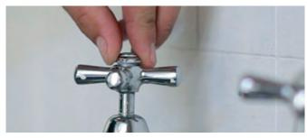
Undo the screw and remove the handle. If the tap has a metal cover, unscrew it by hand, or use a wrench or tap spanner.
