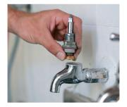
Put the tap back together, turn it off, and turn the water main back on. Check the tap to make sure it's no longer leaking.
