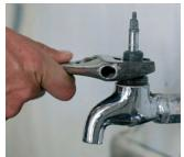
Unscrew the tap bonnet, and completely remove the headgear. You should see a large body washer, o-ring and jumper valve. The jumper valve should fall out.
