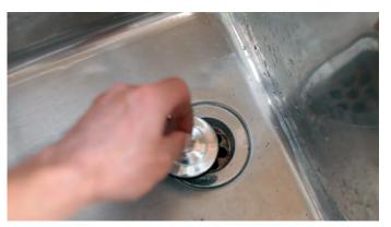
Turn on the tap to release any water left in the pipe, then put a plug in the basin to stop any parts falling down the drain as you work.
