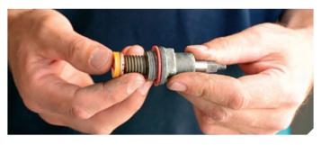
Refit the bonnet and spindle. Be careful not to over-tighten the nuts.
